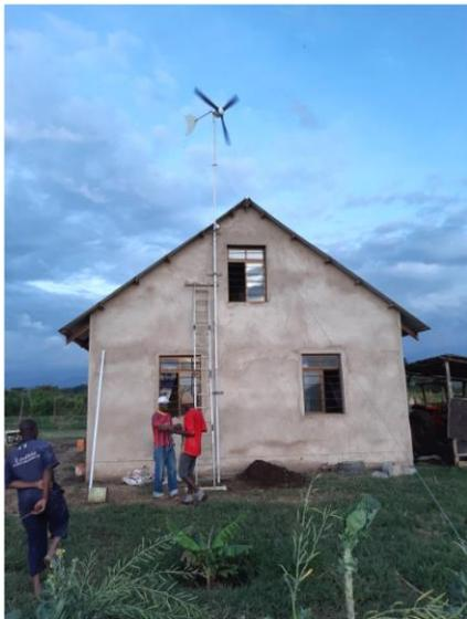
It is a modest 2 story building with 4 sleeping rooms. A windmill and solar panel provide current .By means of an inverter the current is converted to 220 V for light and charging cell phones.
